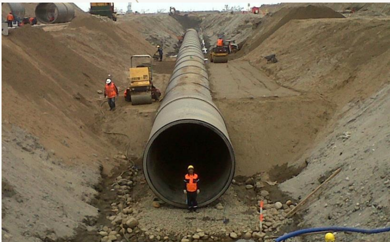
Sewage outfall of La Taboada (Lima, Peru). I.D.= 3.000 mm
