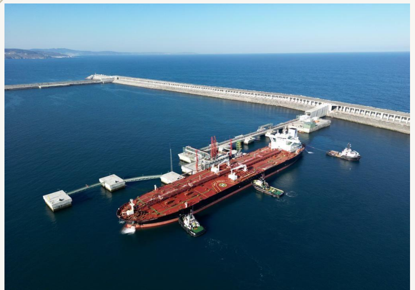
Crude oil unloading jetty in the Port of Langosteira (Spain)
