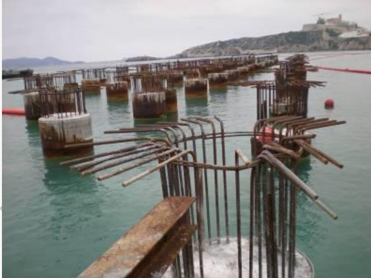
Extension of the Port of Ibiza, Balearic Islands. (Spain)
