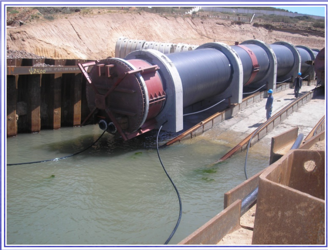
Beni-Saf (Algeria) desalination plant launching ramp for pipeline I.D.= 2.400 mm
