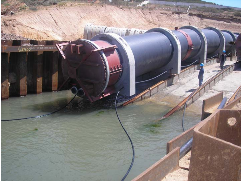
Photo 3: Introduction of the pipes in the sea: Beni-Saf
