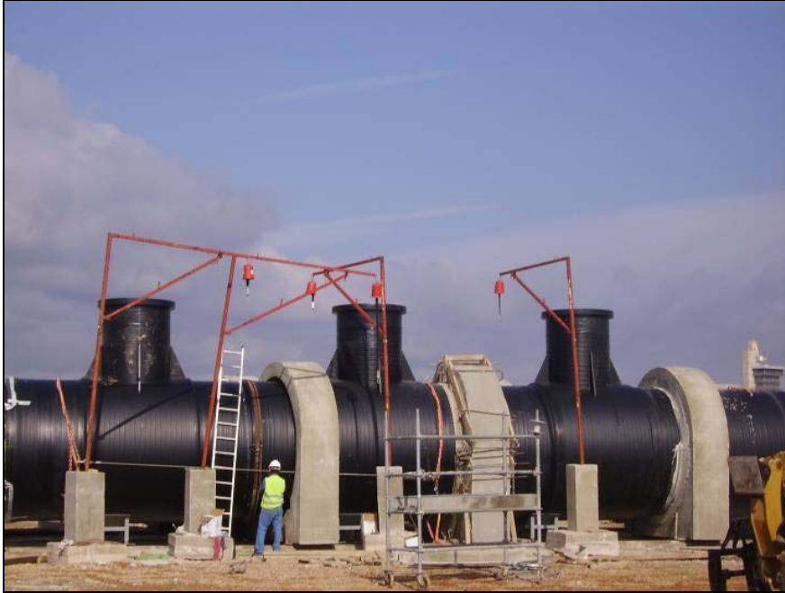
Figure 3 Algeciras outfall (diffuser zone), during ballasting
