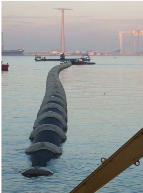
Figure 2. Cadiz outfall of 1800 mm, during sinking
