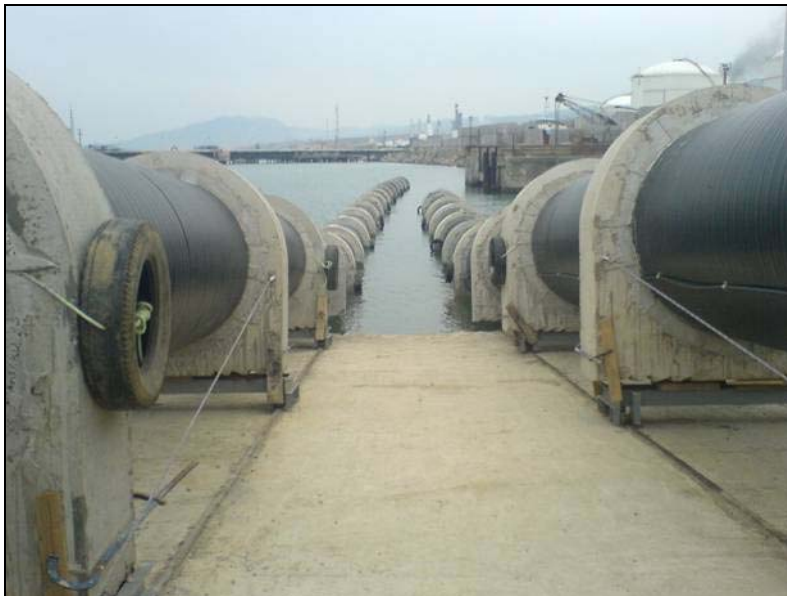
Figure 8 Skikda: pipes during launching at the port
