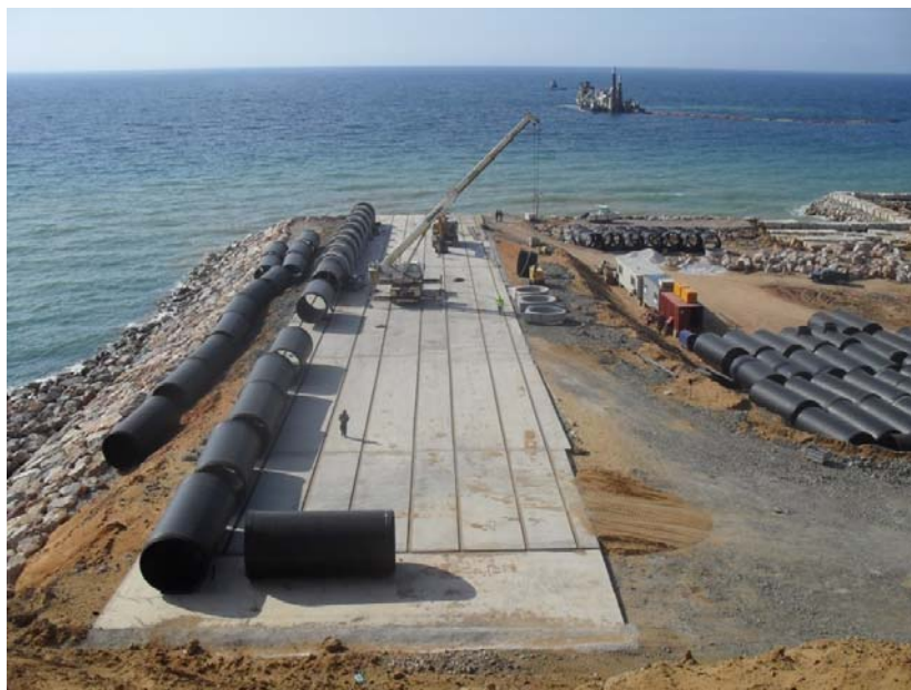
Figure 6 Works on land at Koudiet.
