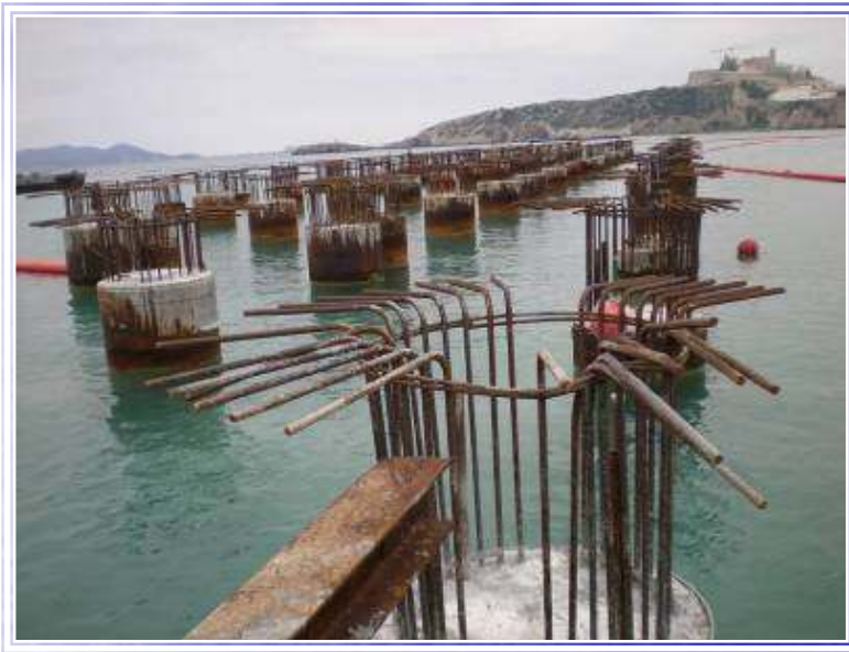
Extension of the Port of Ibiza (Balearic Islands), Spain
