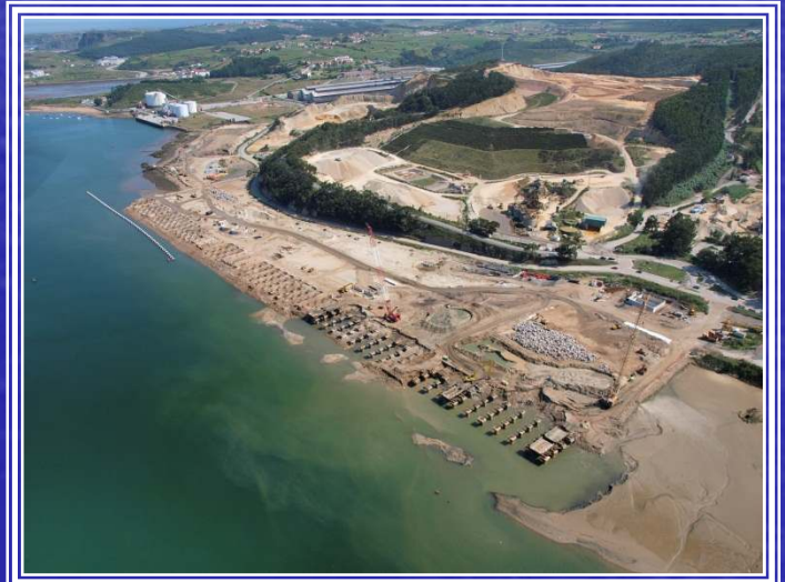
Extension of the port of Aviles along the right bank, Spain
