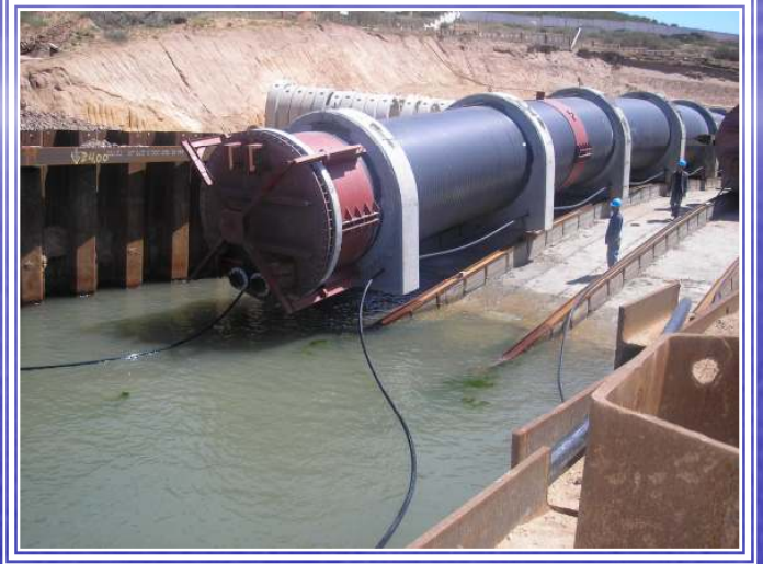
Beni-Saf (Algeria) desalination plant launching ramp for pipeline I.D.= 2.400 mm
