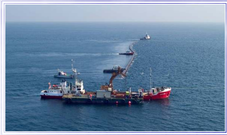
Sewage outfall O.D.=1.600 mm of Berria (Santander, Spain)
